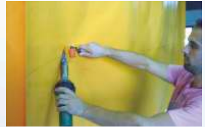
Repairing the Duct
